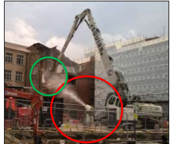
Above – showing mistlers being used to dampen down dust
