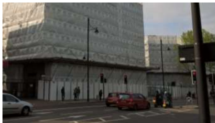
Above – hoardings at street level and protective sheeting above
