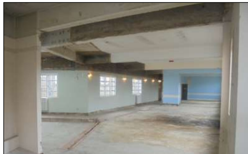
Above – showing internal 'strip out' works in the Town Hall
