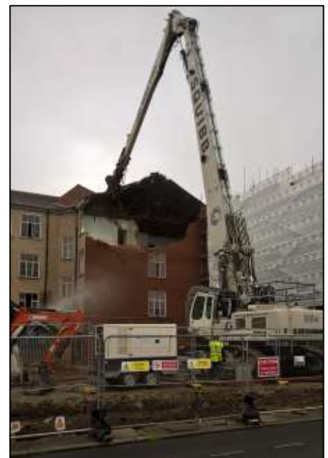
Above – ‘Long range Excavator’ used for demolition
