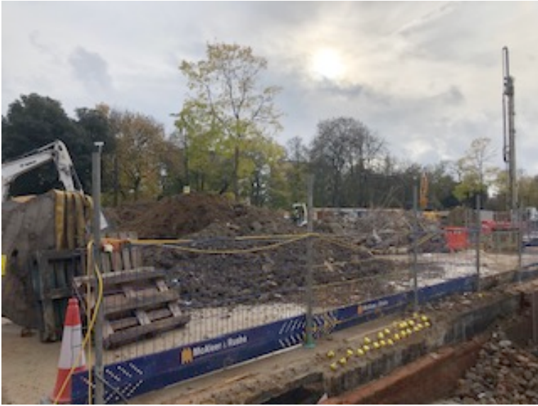
Excavator on site moving materials
