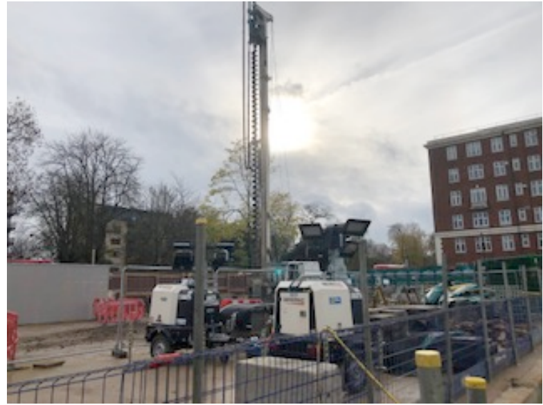
Auger Piling
