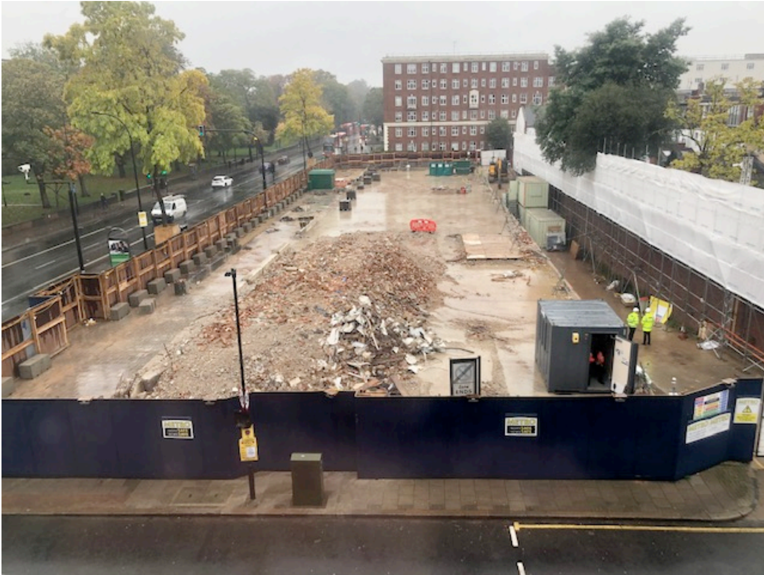
Arial view of the site, minimal construction
