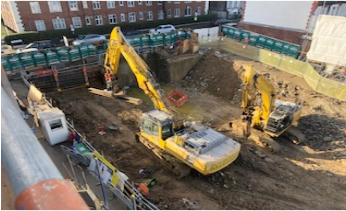
Shoring up of the basement using the excavator
