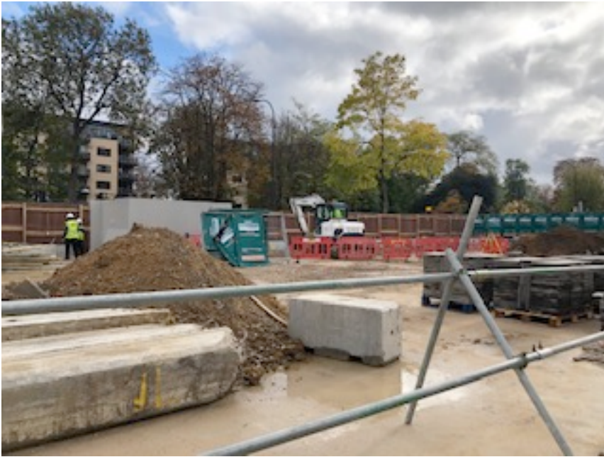
Excavation and Pile Probing Works
